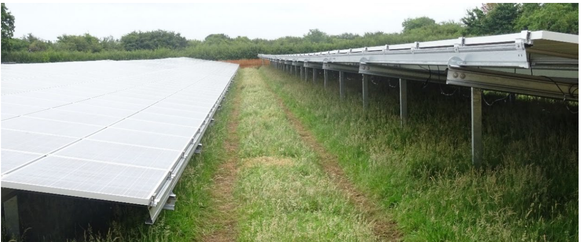
Photograph 14.14: After Solar PV Panels Bolted-on (Bentham Farm, August 2015)
