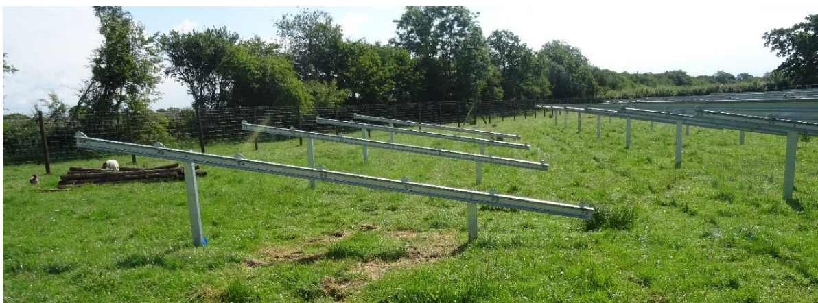
Photograph 14.13: Mounting structures Installed (taken at Bentham Farm, July 2015)
