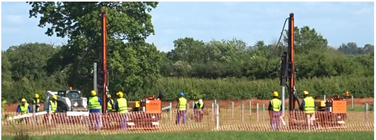
Photograph 14.11: Mounting structures being Installed (Bentham Farm, July 2015)
