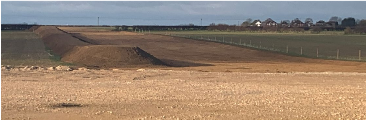
Photo 14.22: Example of Topsoil Stripped Before Trenching Starts
